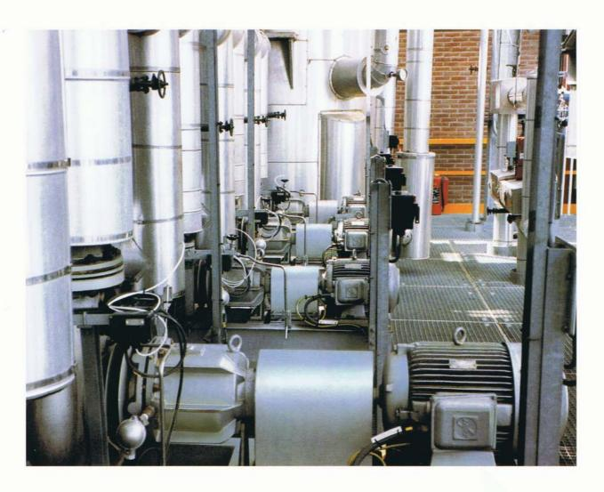
Hot Oil Circulation Pump with magnetic coupling
