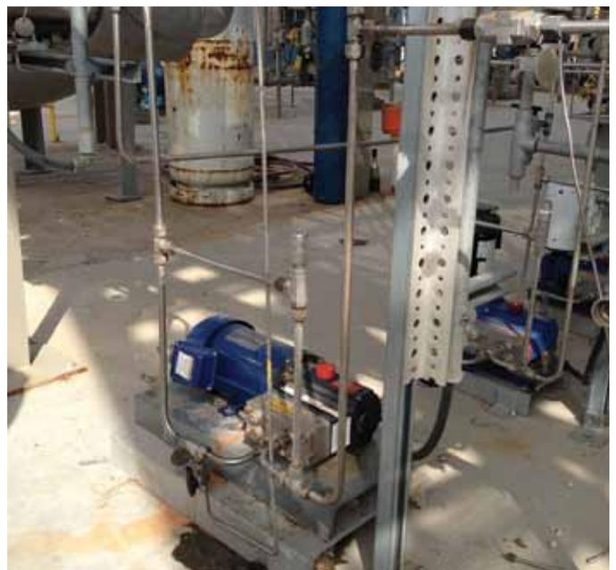
Hydra-Cell pumping ethanol-based liquid for making jet fuel.
